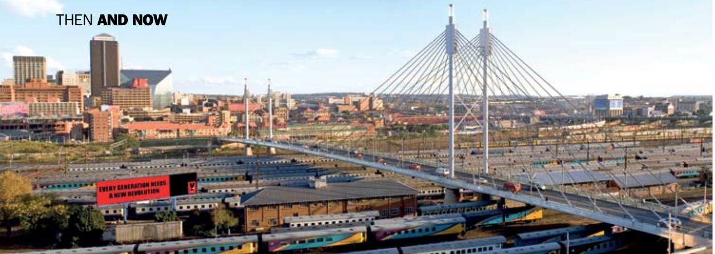
Above: The Nelson Mandela Bridge crosses the Johannesburg Station shunting yards, linking the business districts of Braamfontein and Newtown Below: Civil engineers survey road infrastructure in Pietermaritzburg
